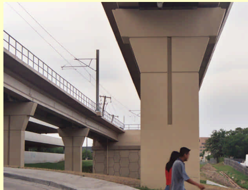
Massive support columns
