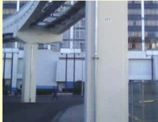
Massive support columns
