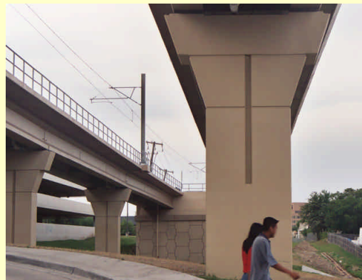
Massive support columns
