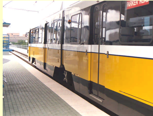
Open Passenger Platforms
