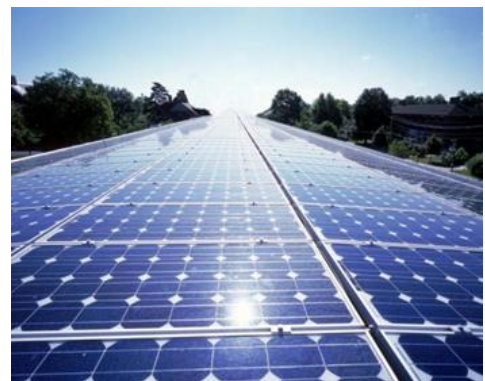
PV Solar Panels Covering Roof of Toll Road.
