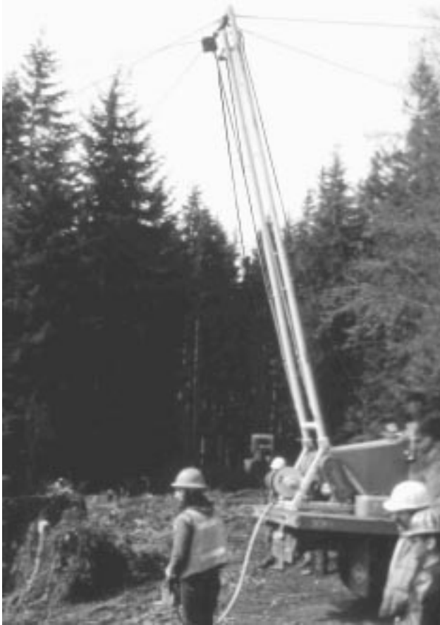
Figure 21 — Small, highly mobile cable yarders can provide economical yarding of smaller logs on steep ground with minimal impacts.
