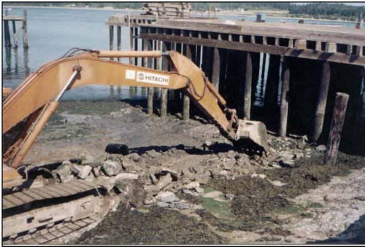
Figure IV.7. Track-hoe removing rubble during low tide.
