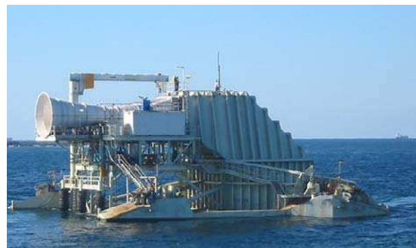
Terminator (Energetech Oscillating Water Column)
