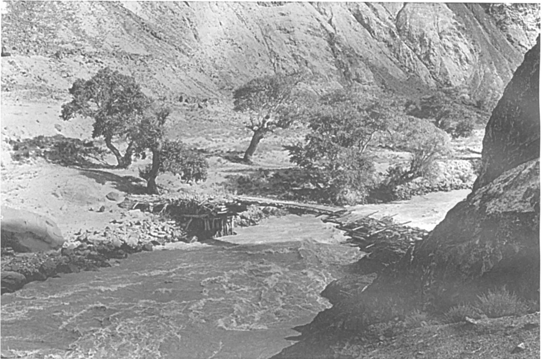
PLATE VI Cantilever bridge, Karatash River valley, south of confluence with Kaying, August, 1996
