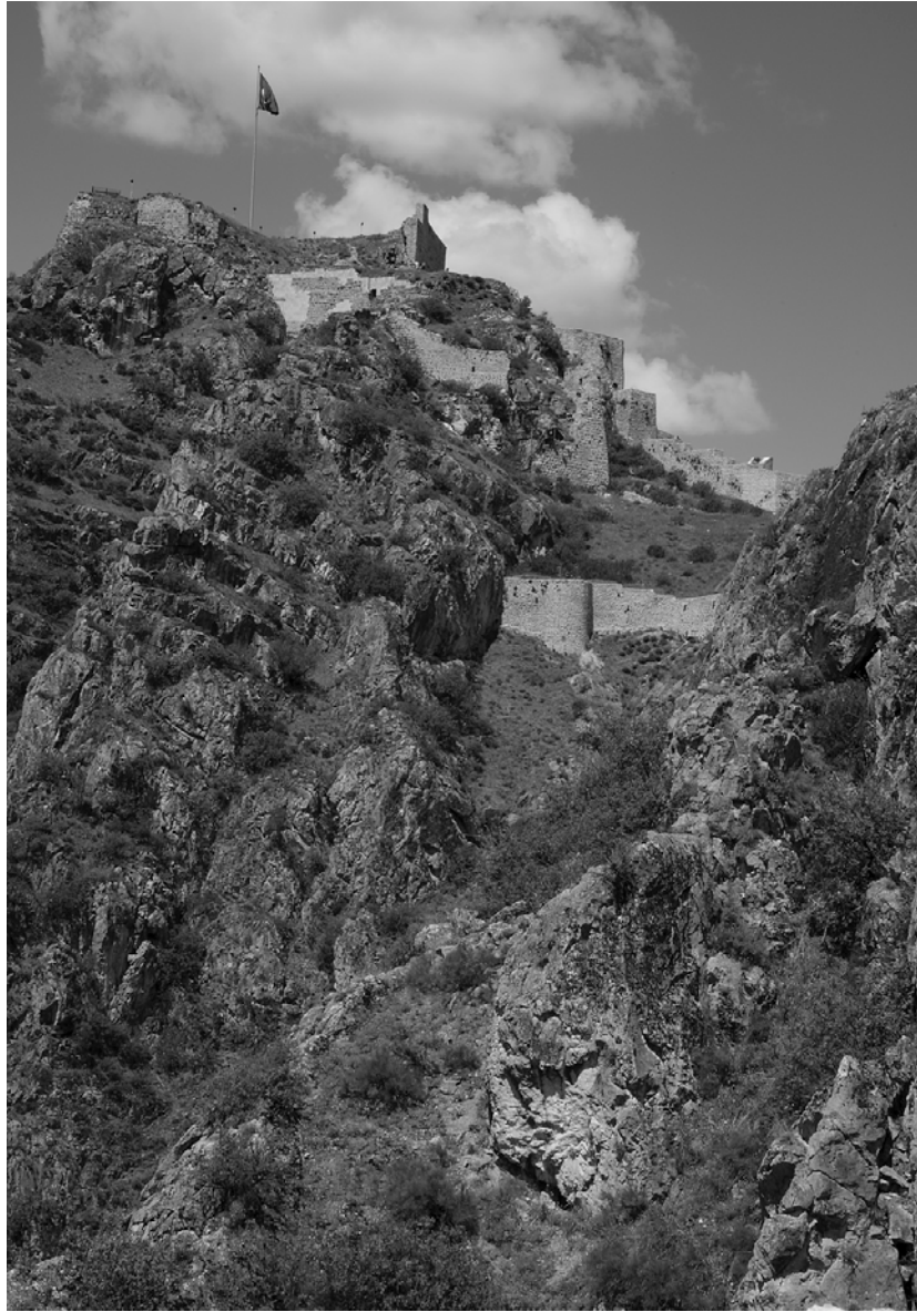
FIG. 4. THE FORTRESS WHICH LOOMS OVER HISTORIC AMASYA, MUCH REBUILT OVER THE CENTURIES AND RECENTLY RESTORED. PHOTO JUNE 2014
