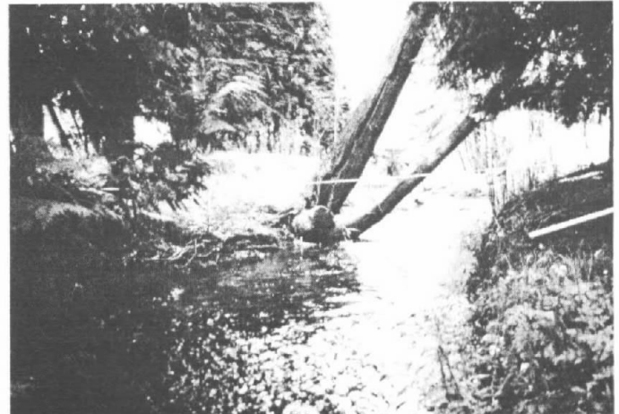
Figure 2d. Completely Unstable Reach (I). Minimal bank vegetation and nearly vertical, severely eroded banks. The right bank (left in picture) has been eroded back far enough to almost undermine the large tree (Thornton Creek, Site T1).
