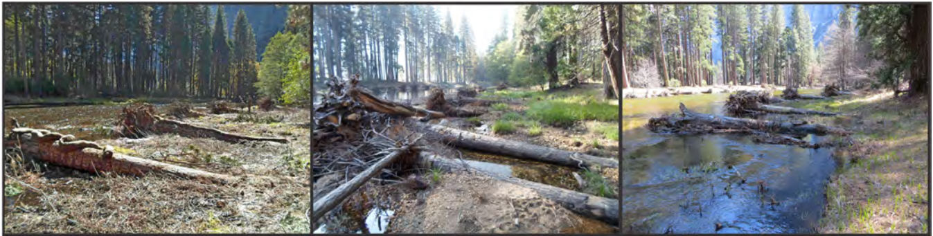
FIGURE 8 Photographs taken over a three-year period of the channel-narrowing and riparian-restoration project constructed about 200 m downstream of Ahwahnee Bridge along the right bank of the Merced River. Project consists of logs with root balls placed perpendicular to the bank, designed to trap bedload sediment and promote riparian vegetation growth. Image dates October 2016 (left, just after project installation), October 2017 (center), and April 2019 (right; higher discharge at this time, inundating the foreground sediment). Note the lack of significant sediment accumulation between the log structures. An additional project constructed September 2017 is visible cross-river in the last two images [Color figure can be viewed at wileyonlinelibrary.com ]
