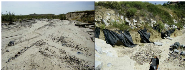
Figure 4 Views upstream (left) and downstream (right) of Borrego Canyon (Irvine, CA, USA)
