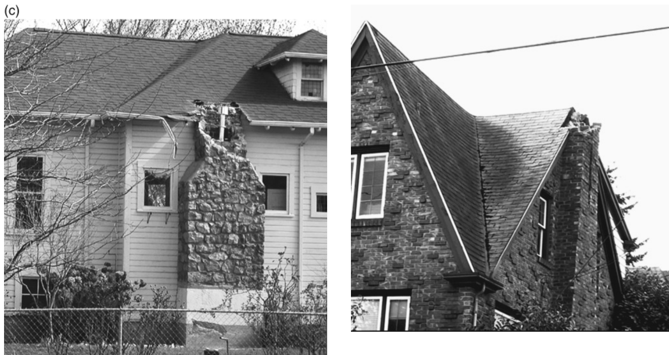
Figure 4. (a) Examples of class 1 chimney damage (the right-hand image also shows a class 2 damaged chimney on the right side of the house). (b) Examples of class 2 chimney damage. (c) Examples of class 3 chimney damage.
