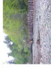
East beach historical bulkhead buckles under pressure from hillside.
