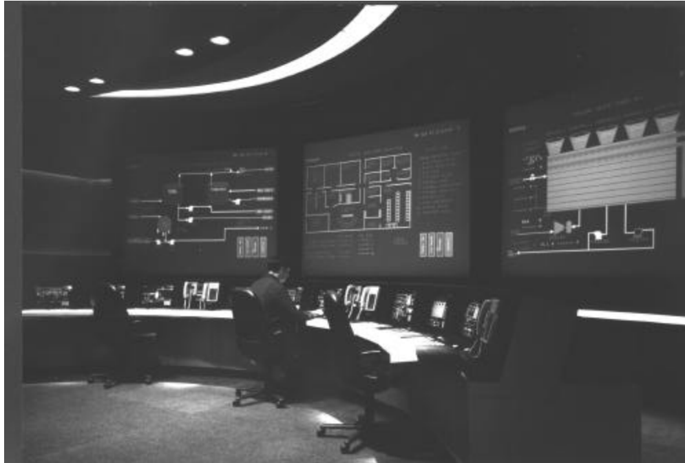
Figure 2.5 Photograph of a control room for a DCS. Courtesy of Honeywell.
